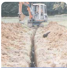
Ground loop in trench
