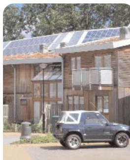
PV roofs on ecohomes
